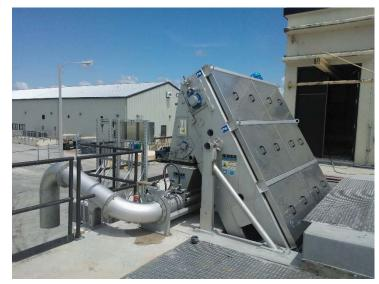
allowed upstream water to escape over the weir. All 90 MGD had to face the EscaMax and leave their baggage behind on the screen where it was efficiently removed, washed conveyed and compacted.
