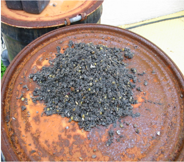
Existing Grit System
