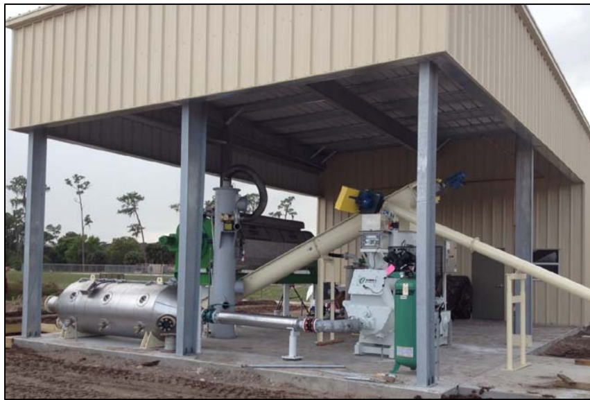
Facility Under Construction - Small Footprint
